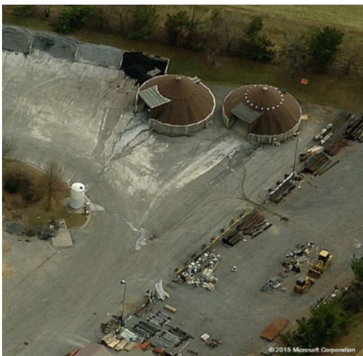
Current Frederick storage (at Public Works dept. 111 Airport Drive East).
