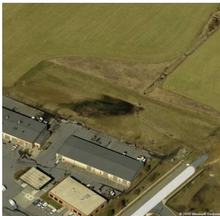
Current stormwater control on that property.
