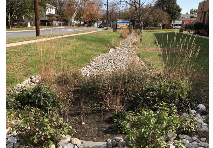
Newly added rain garden to address drainage issues
