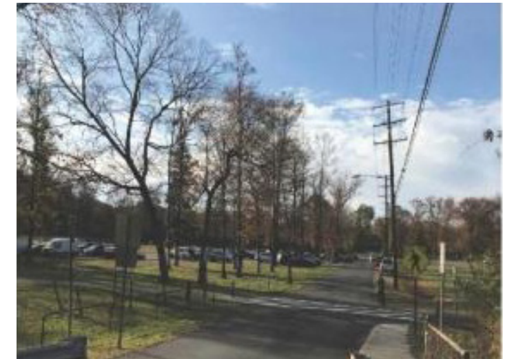
Water pools near parking
