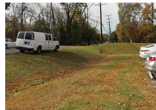
Ditch by parking lot
